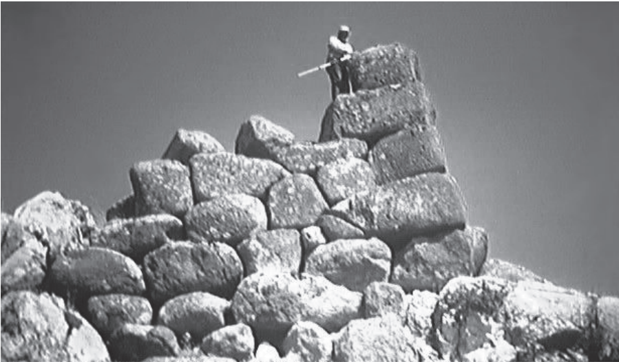
Expedition director Stephen Lumsden holds surveying target on remains of the southeast corner of the cyclopean retaining wall at Gavurkalesi. The andesite stones which make up the wall were quarried about a mile away. (Photo taken Sept. 1994)
